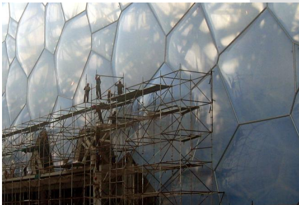
Figure 67 –Image showing the installation of ETFE sheets over the structure..
