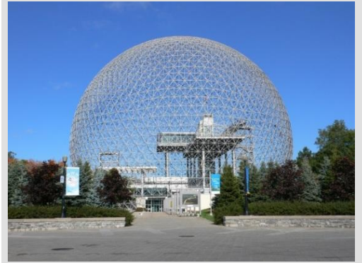
Figure 24 -The Geodesic Dome (1967) in Montreal by Buckminster Fuller comprises three quarters of a geodesic sphere. The outer Hull is made out of triangles and is linked to the inner hull consisting of hexagons.
